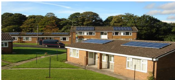
Photo showing: two systems on semi-detached bungalows (foreground), four systems on a block of flats (background right) and a further three bungalow systems (background left)
