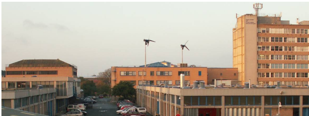
The two turbines are mounted on the roof of the college Innovations Centre building
