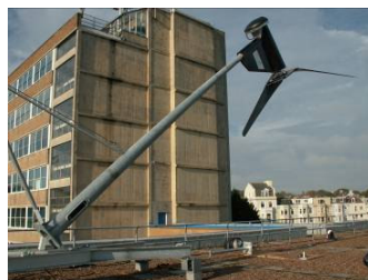
Installation of one of the turbines
