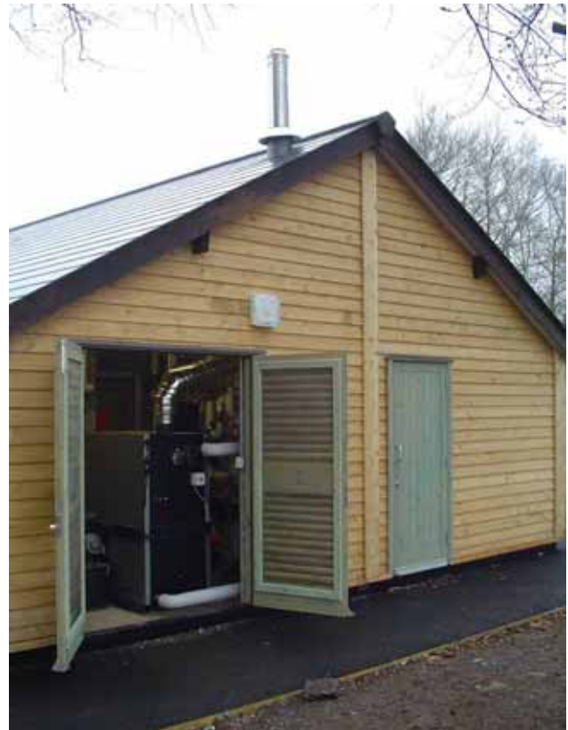
The boiler room and fuel store (right)
