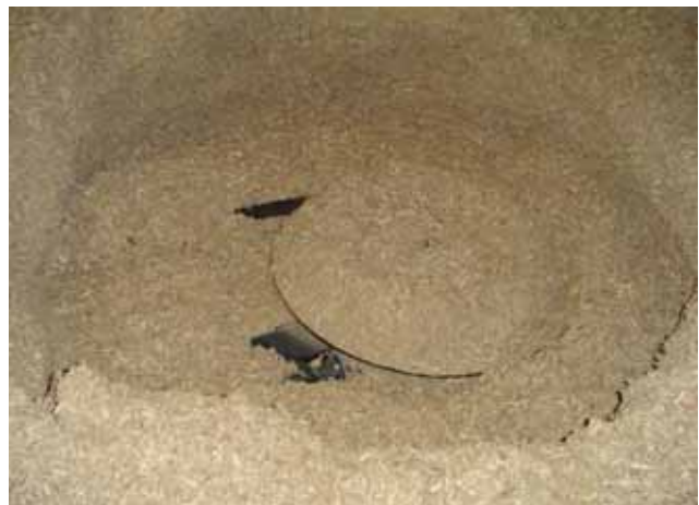
Spring-arm outfeeder within the fuel store
