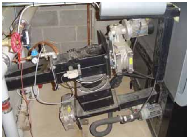
Fuel feed (from left), with failsafe fire flap, and auto-ignition system (bottom right)
