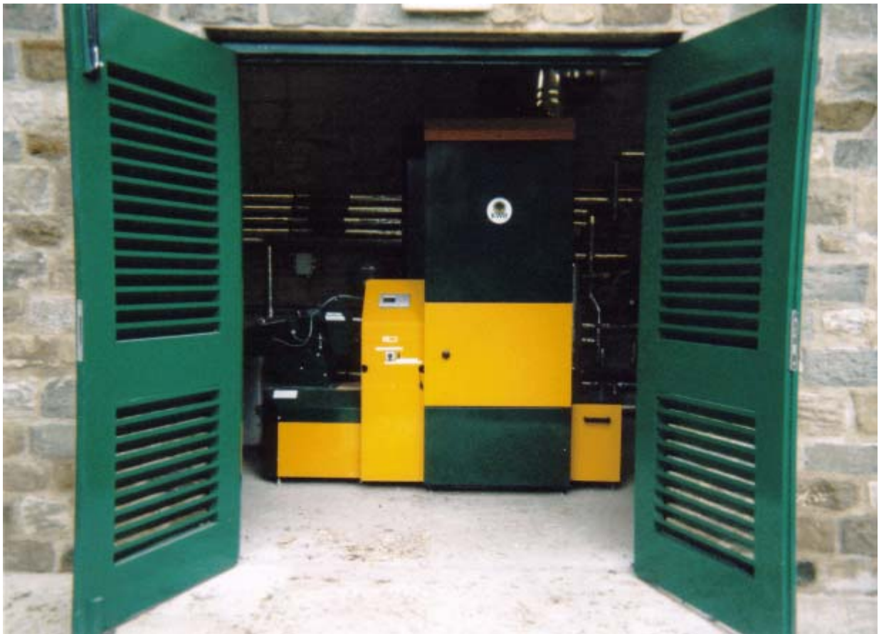
KWB USV D 100 kW automatic woodchip boiler, fuel feed from left, ash bin on right
