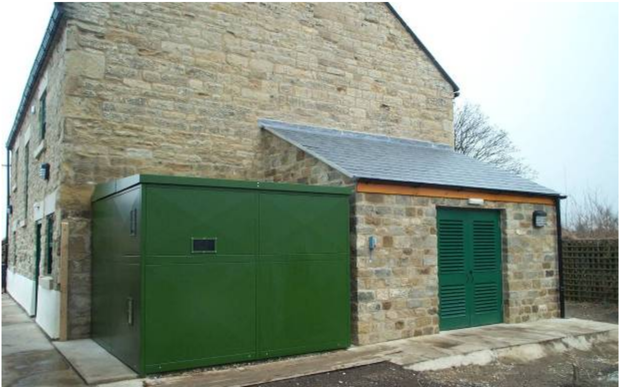
The boiler house and woodfuel hopper
